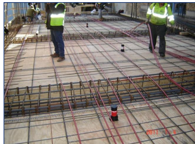
Figure 12: Post-Tensioning Installation on the New Addition; Picture Courtesy of Luis Ortiz
