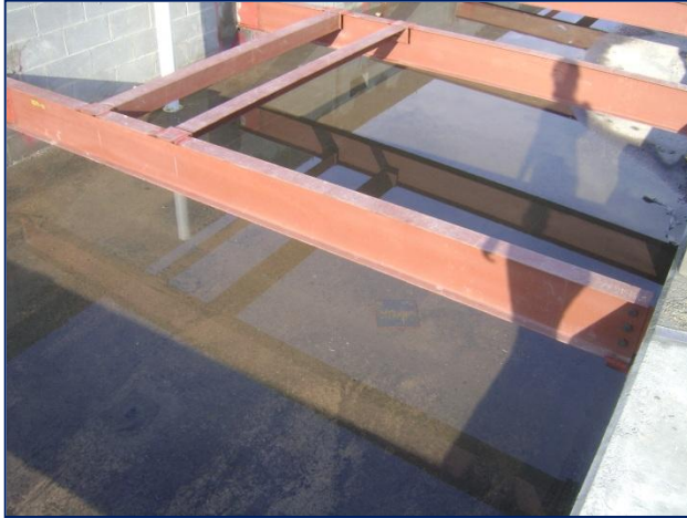
Figure 8: Pooled Water on Existing Roof; Picture Taken by Clara Watson
