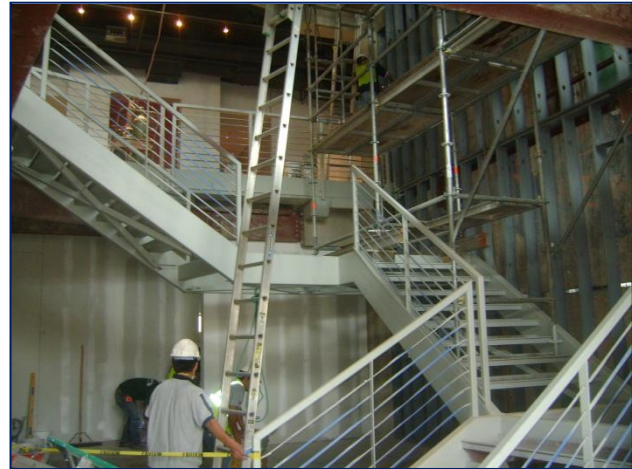
Figure 11: Scaffolding and Signature Wall Installation; Picture Taken by Clara Watson
