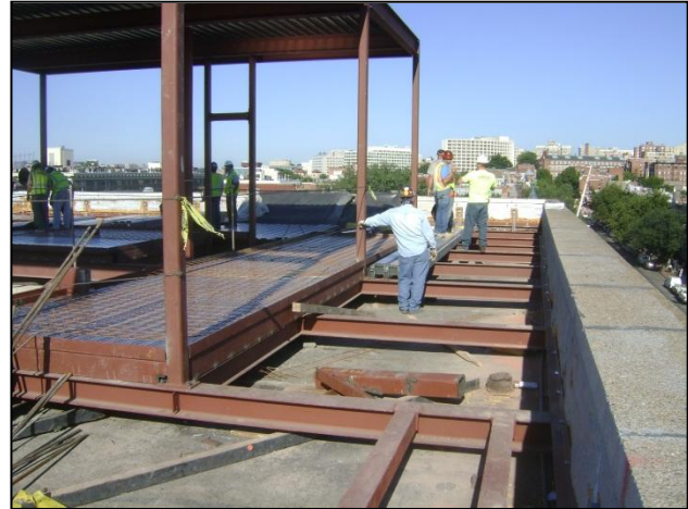
Figure 6: New Roof Constructed Over Existing Roof, Picture Taken by Clara Watson
